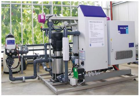
A Priva Vialux Ultra Violet sterilisation unit that allows sterilisation of collected drain water, which in turn is stored in a 'clean' tank before being recycled to the crop.
