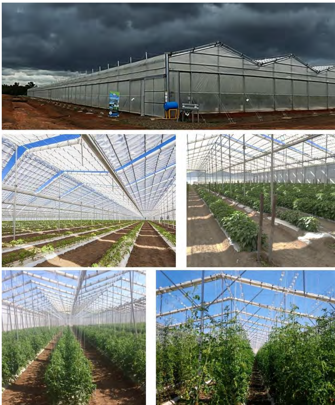
Figure 10. Examples of retractable roof structures with peaked roofs. There are also models with flat roofs used in overseas regions where rainfall is low. A commercial retractable roof structure in Bundaberg was setup in 2015. Four extreme weather events (storms with intense wind and rainfall) between 2015 and 2017 demonstrated the level of protection that these structures can provide to vegetable crops (tomatoes and capsicums). On sunny days, the roof can be opened totally or partially to modify solar radiation, soil and crop temperatures, and air relative humidity. Similar structures have been operating in warm climates such as Florida, USA, Mexico, South Africa and Turkey (Image source: (Images source: DAF and < https://www.cravo.com >).
